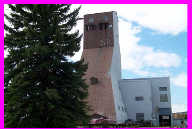
The mine's 5,000 foot vertical shaft elevator house
