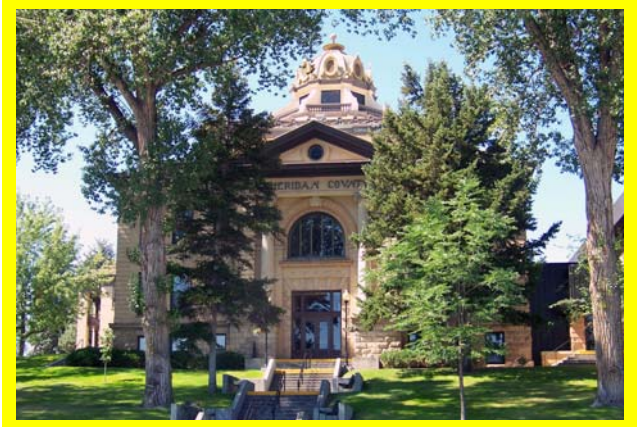
The historic Sheridan County courthouse
